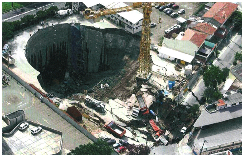
Above: The Pinheiros station cavern and shaft collapse in Sao Paulo in January 2007
