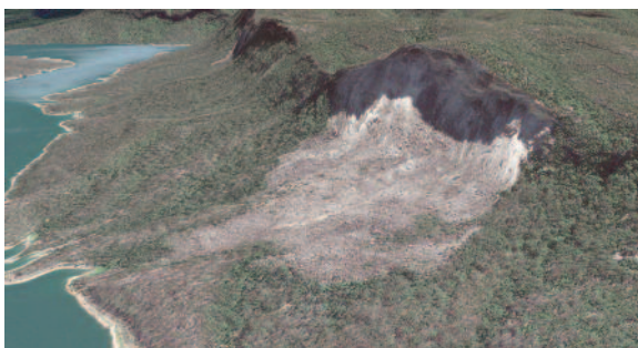
Figure 6 Collapse at Nattai North
