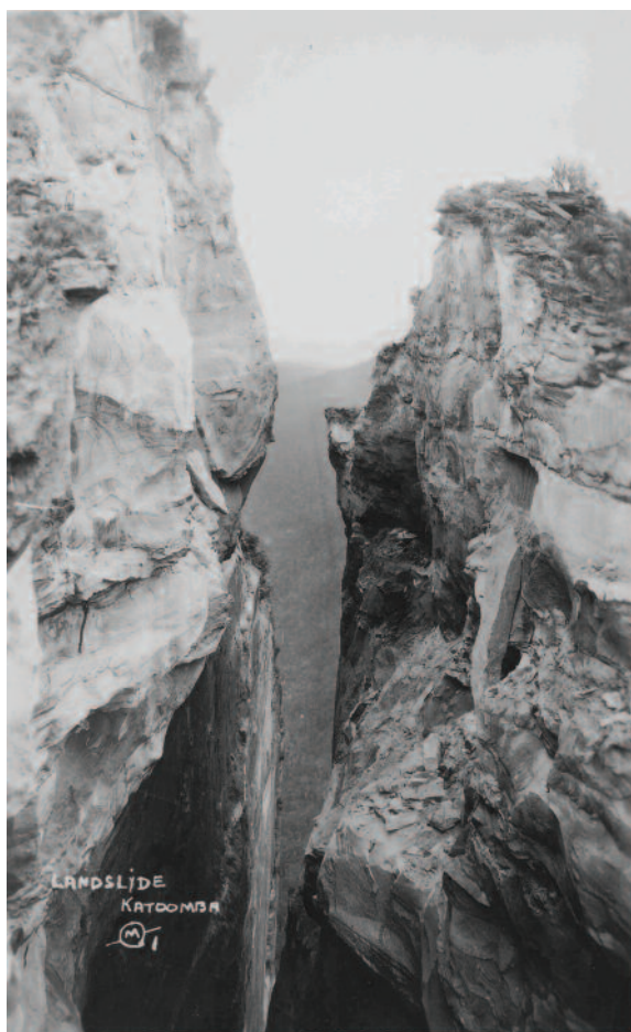
Figure 3 Tension crack at Dogface Rock, Katoomba, January 1931
