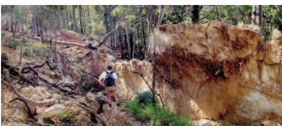
Figure 7 Slope failure in Sugarloaf State Conservation Area, late 2013
