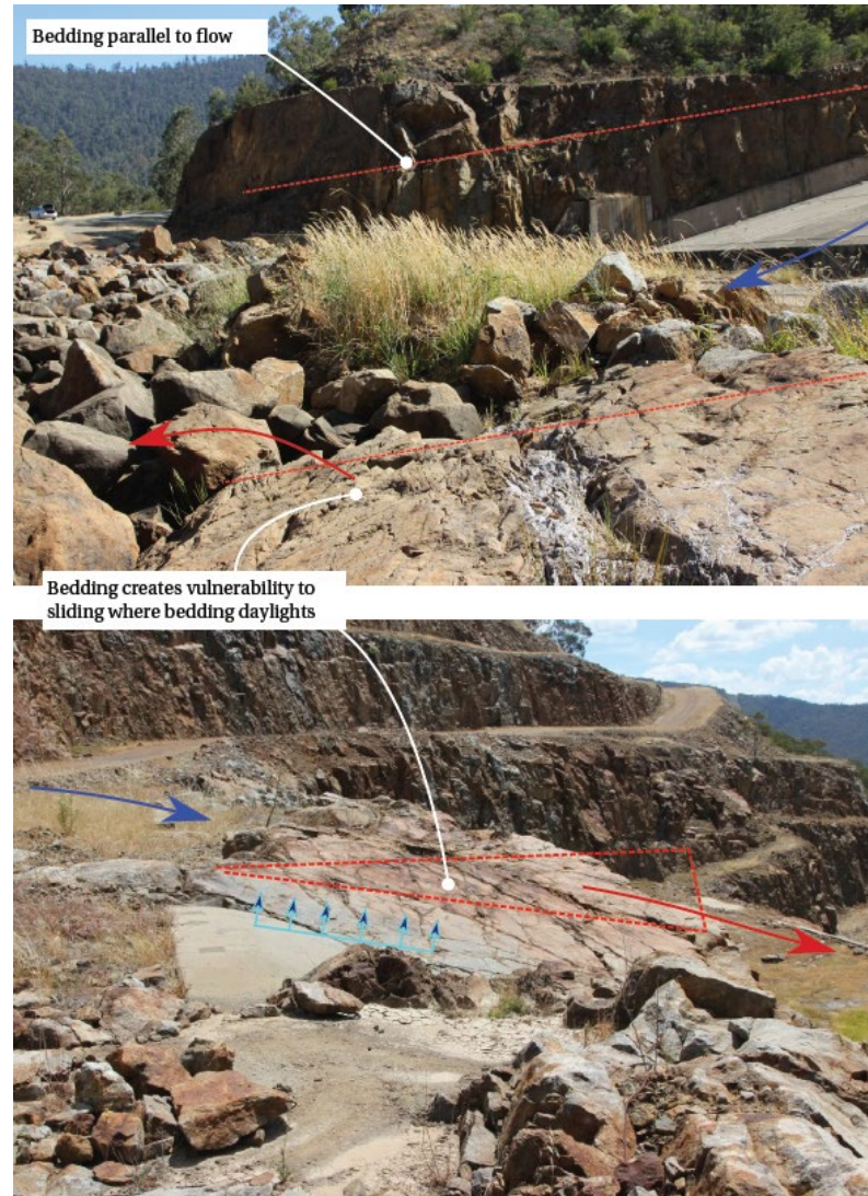
Figure 3.36 Dartmouth dam - persistent planar beds parallel to flow direction
