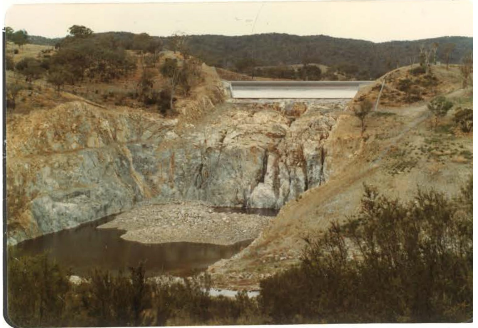
Spillway after initial operation.
